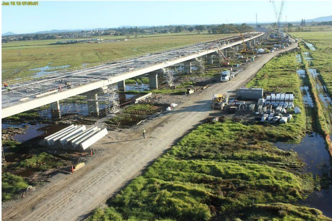
Kempsey bypass under construction.
